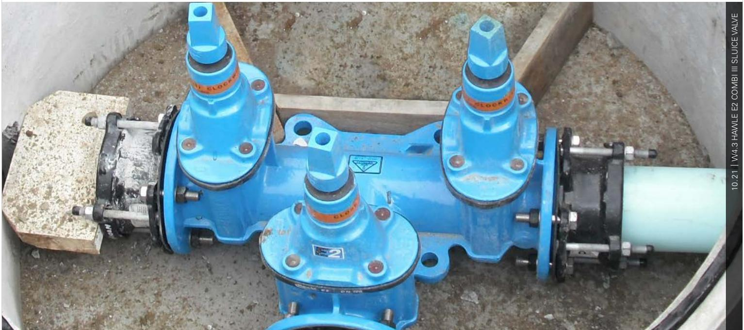
10.21 | W4.3 HAWLE E2 COMBI III SLUICE VALVE
