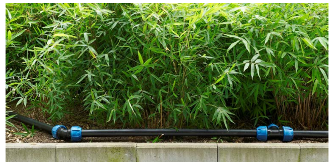
FIG. 1 Photos of the Compression Joint installed
