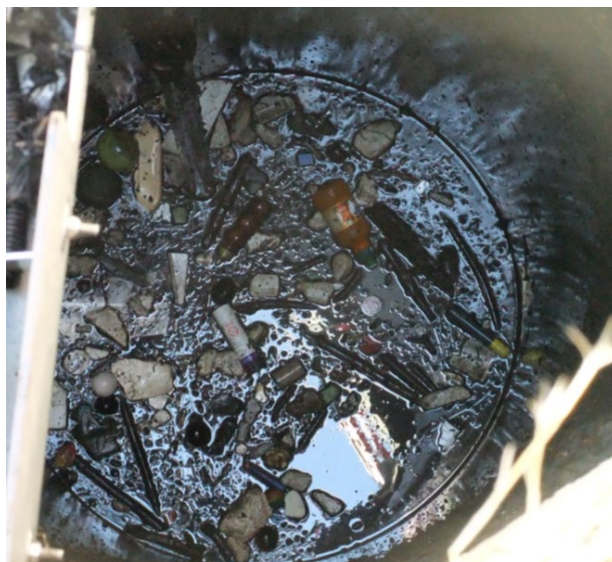
FIG. 4 View of floatables and oil collection zone
