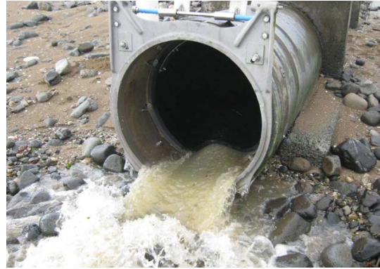
FIG. 13 DN600 – Te Puru Boat Ramp, Thames
