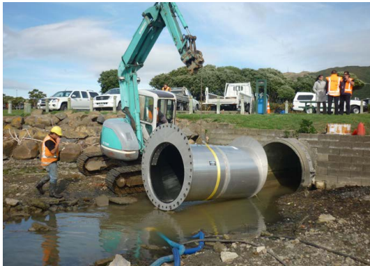
FIG. 10 DN900 Valve in DN1350 pipe, Porirua
