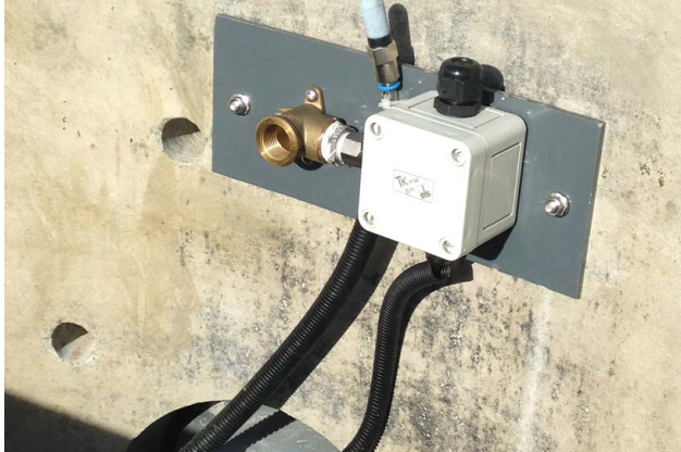
FIG. 2 Internal relay box
