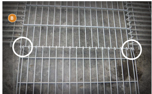
FIG. 5 Outer hook fitted
