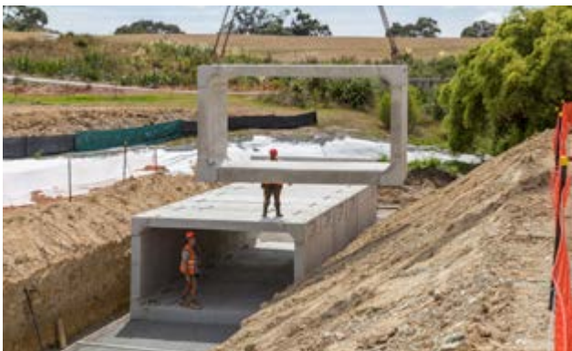
FIG. 5 Place first culvert into required position
