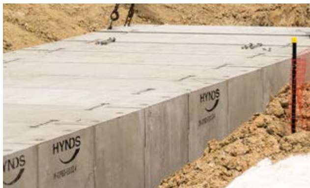
FIG. 8 Fill recess with Sikagrout 212 or equivalent.
