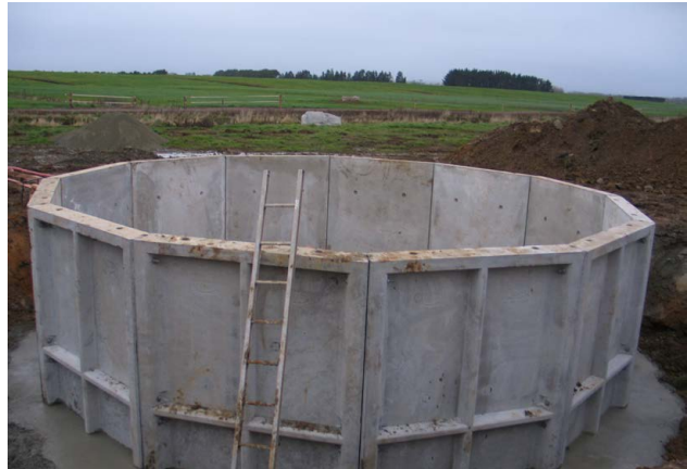
FIG. 3 Hypond ready for placement of back fill
