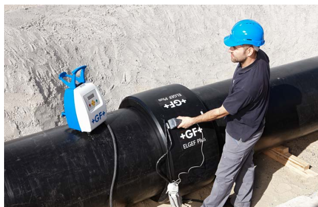
Electrofusion Jointing of PE Pipes and Fittings for Pressure Applications.
