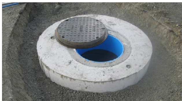
FIG. 2 Precast Concrete Slab and Class D Cover
