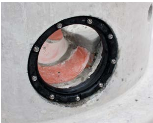
FIG. 3 Hyseal ready to connect pipe
