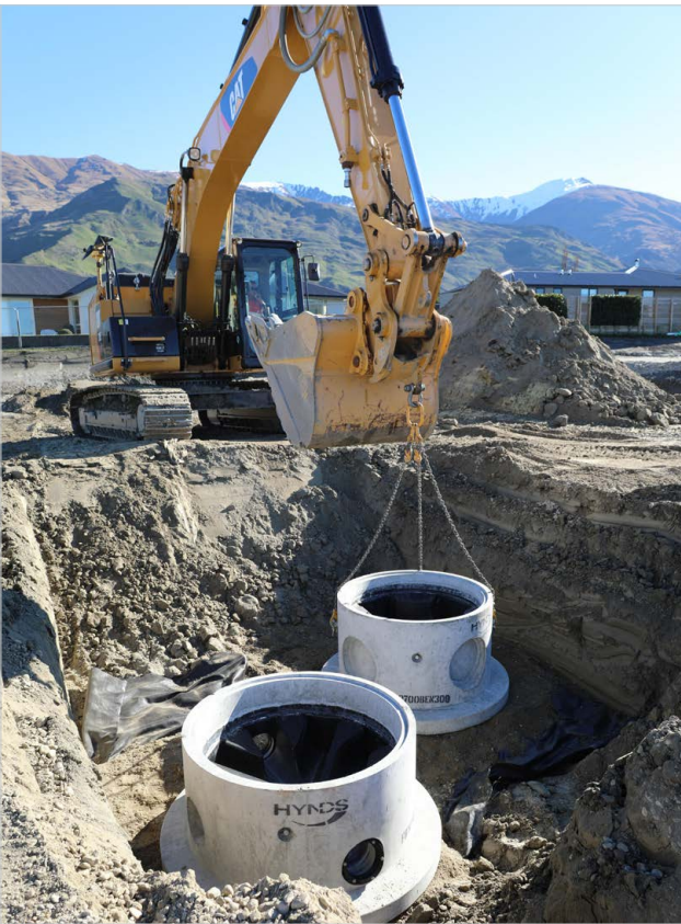
FIG. 8 Hybencher installation in Cromwell
