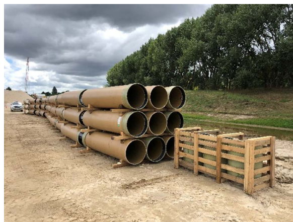
FIG. 10 Stacked pipe (DN600) stored on timber dunnage and fittings stored in timber crate
