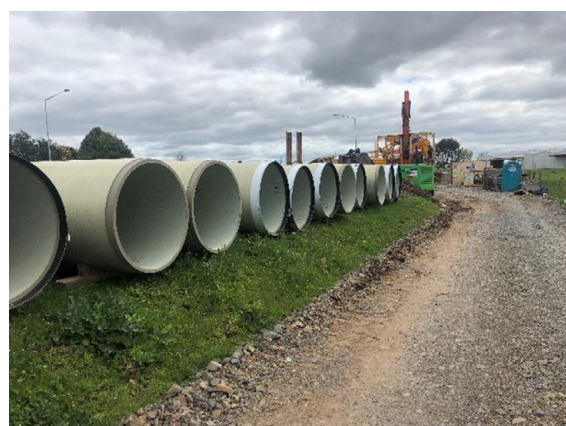
FIG. 11 Large diameter pipes stored on site on timber dunnage
