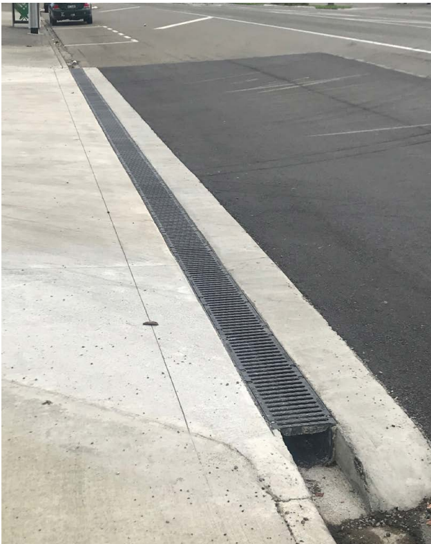
FIG. 1 Service Station, Sanson
