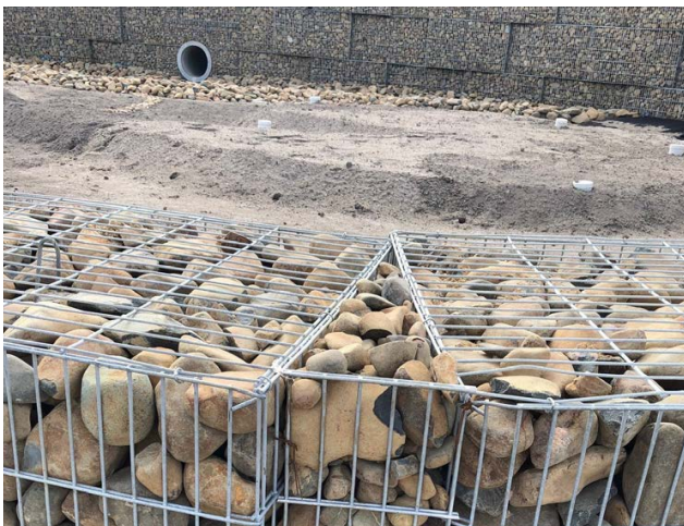
FIG. 1 Rawe Stonebox using Mangatangi Stone (Refer Table 2)
