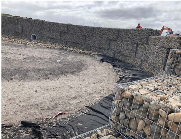
FIG. 1 Rawe Stonebox using Mangatangi Stone (Refer Table 2)
