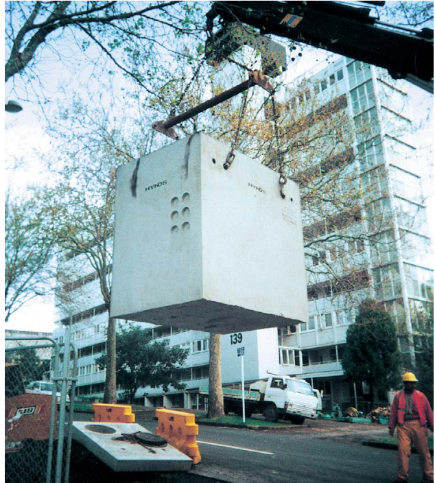
FIG. 1 Concrete Access Chamber being lifted into position
