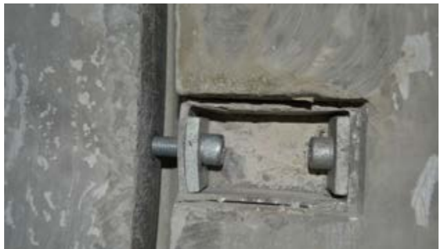
FIG. 11 Restraint assembly in extension
