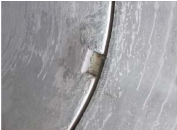
FIG. 14 Restraint box filled with foam & partially epoxied
