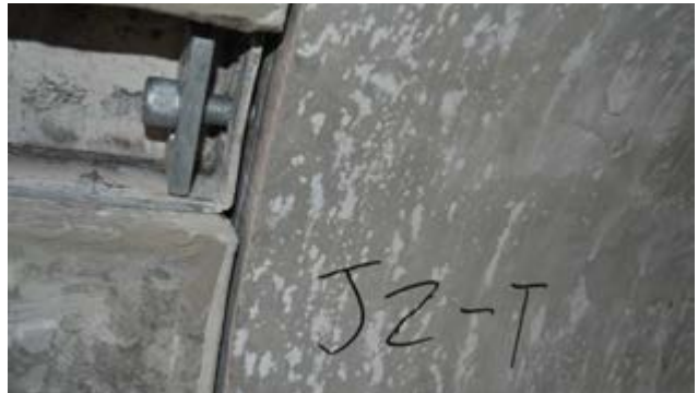
FIG. 9 Restraint assembly in compression
