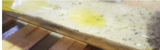
FIG. 1 Concrete Away softened concrete ready for hydro-jetting from drainage pipe
