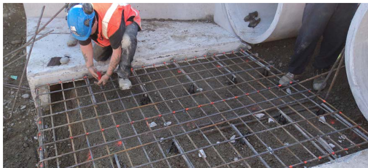
FIG. 4 In situ reinforced concrete
