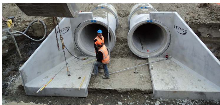
FIG. 3 Multi-Barrel Culvert Wingwalls
