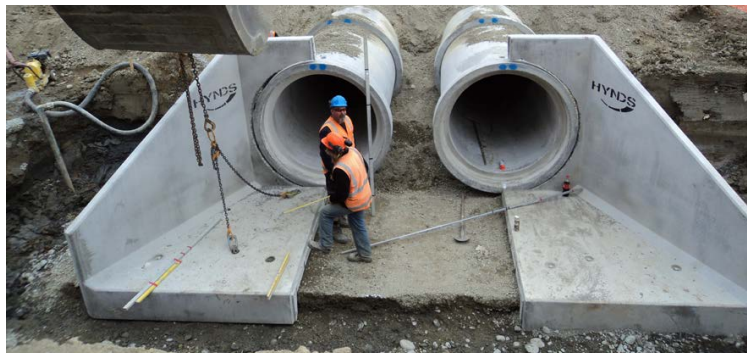
FIG. 3 Multi-Barrel Culvert Wingwalls
