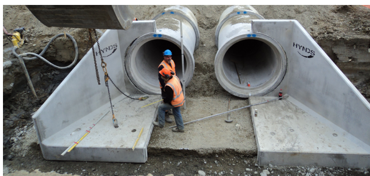
FIG. 3 Multi-Barrel Culvert Wingwalls
