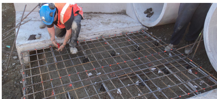
FIG. 4 In situ reinforced concrete
