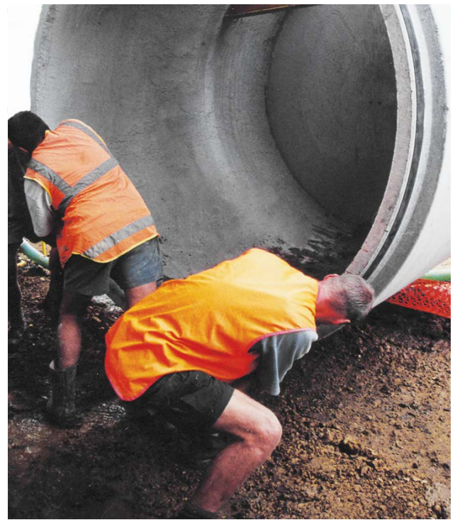
FIG. 1 Ring being placed
