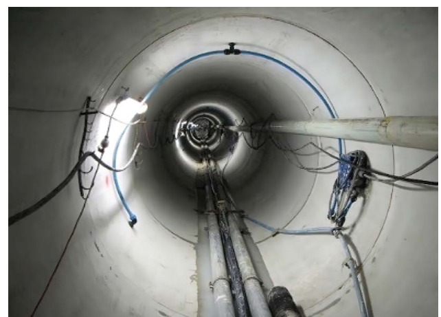
FIG. 13 Image showing grout port connections and drilling fluid pipes and other services.
