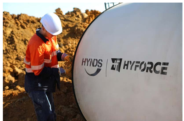
FIG. 6 Installation, fitting and pretensioning of seal rings prior to install.
