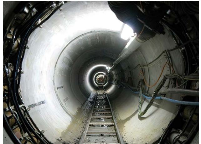
FIG. 10 Typical interjack station illustrating Hydraulic Jacks and Steel CAN
