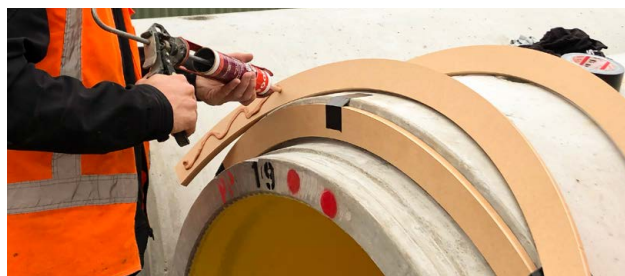
FIG. 7 Showing fixing of MDF packers prior to PERFECT® HDPE lined pipes being installed at Haytons Road Trunk Sewer project, Christchurch.
