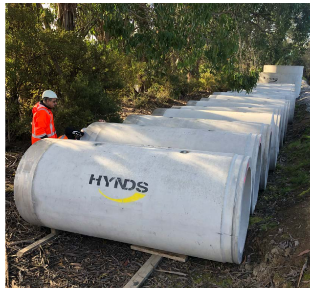
FIG. 14 Typical storage of pipes on dunnage on site.
