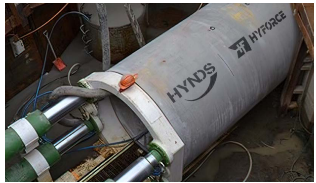
FIG. 3 Typical Hydraulic Jack and Concrete Jacking Pipe being installed.
