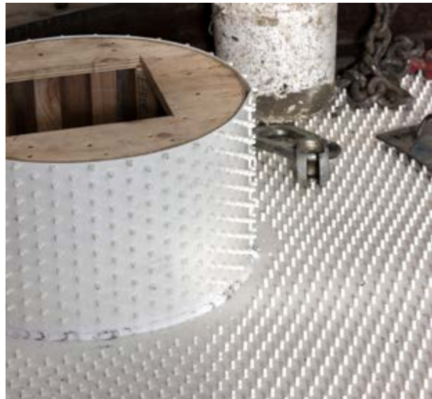
FIG. 14 Liner being installed for a manhole lid
