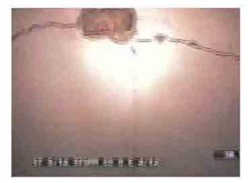
An internal circumferential crack of a DN375 concrete pipe, greater than 0.5mm wide.
