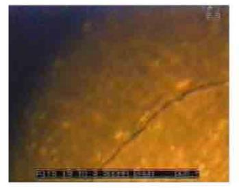
An internal circumferential crack of a DN300 concrete pipe, less than 0.5mm wide.
