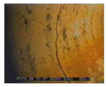
An internal circumferential crack of a DN300 concrete pipe, greater than 0.5mm wide.
