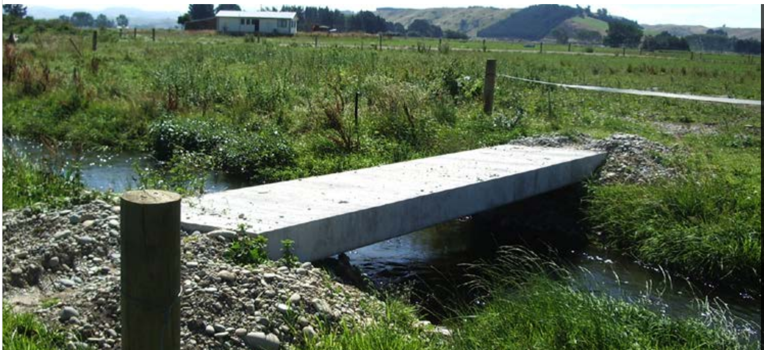
03.15 | RURAL | R4.6 IRRIGATOR WHEEL CROSSING SLAB
