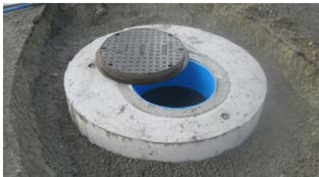
FIG. 2 Precast Concrete Slab and Class D Cover
