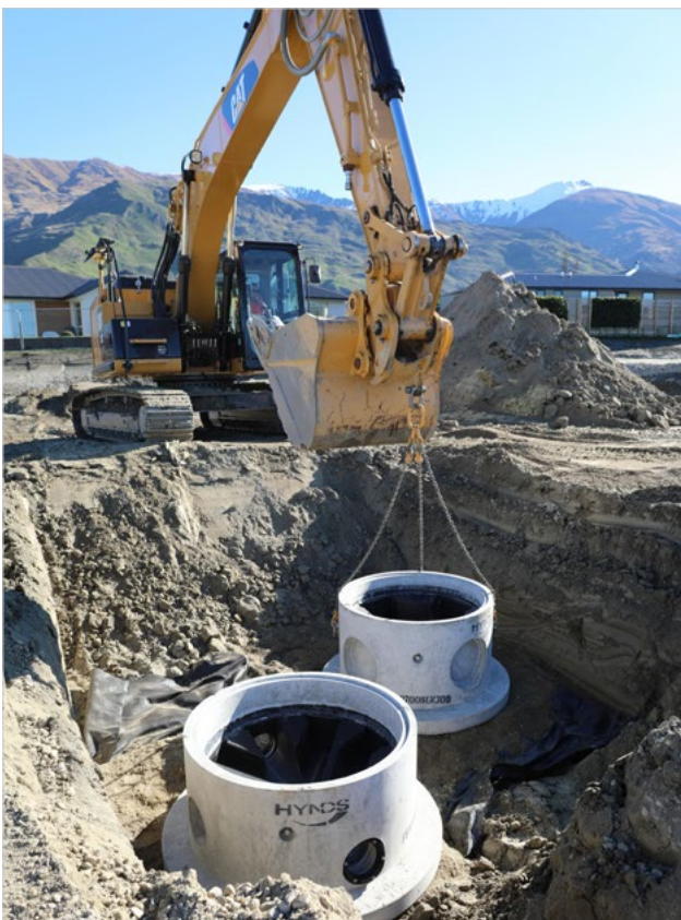
FIG. 8 Hybencher installation in Cromwell
