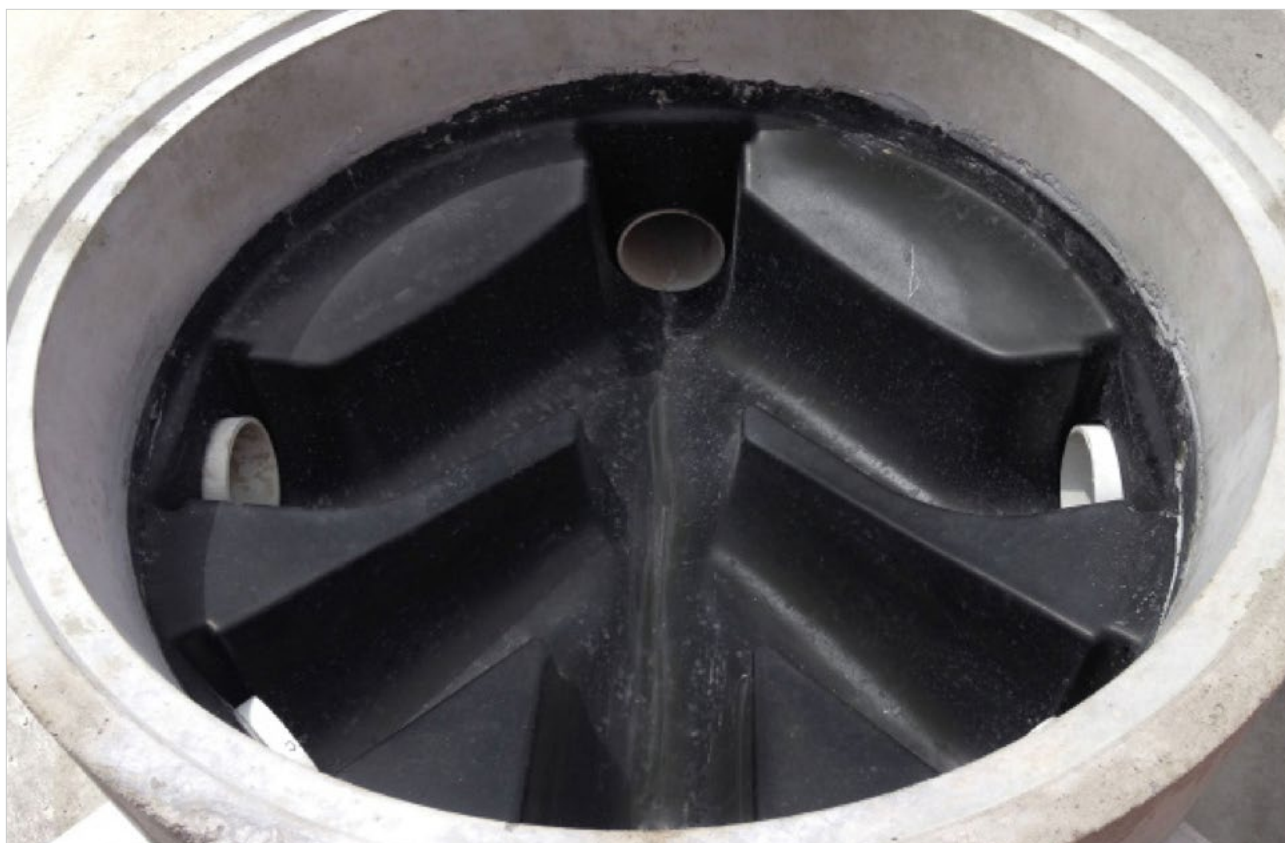
FIG. 5 Detailed view of the HDPE preformed benching of Ø150mm PVC Hybencher
