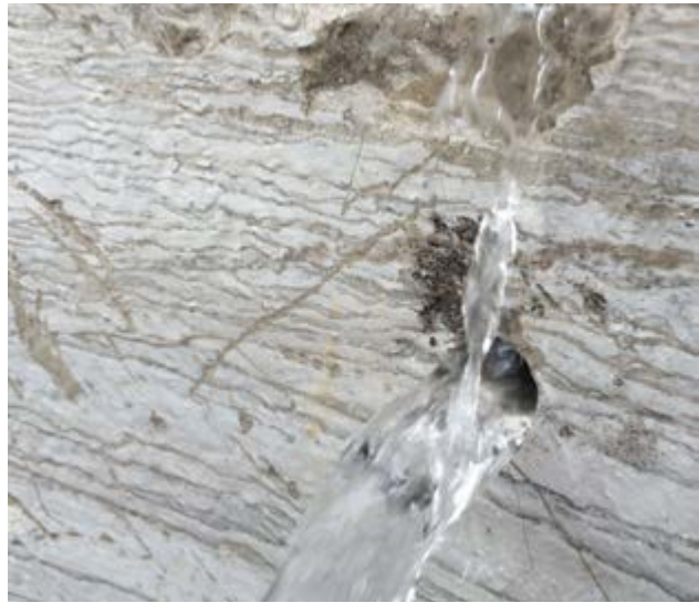
FIG. 1 Leaking MH
