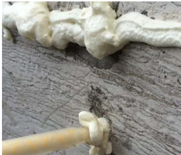
FIG. 2 Aquaseal being applied to permanently stop and seal leak
