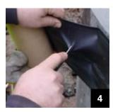
Cut excess material using a knife. Using a rubber mallet or hand held roller, firmly flatten the Aquawrap 360 degrees around joint.
