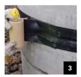
Seal the overlapping area with a 150mm overlap. Be sure not to stretch material at the overlap area.
