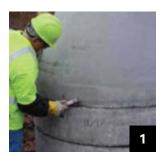
Expose the area that is to be sealed. Clean the entire area around the joint with a wire brush and broom. Remove any sharp protruding edges around the joint with an abrasive tool. When finished cleaning, the entire area must be dry and free of any dirt, grease or oil to ensure good adhesion.
