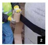
Remove the first foot of paper backing from the mastic. Centre and place the Aquawrap around the joint. Continue to remove paper backing as you apply the Aquawrap to the entire structure.
