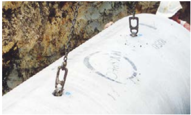
FIG. 6 Pipe is positioned into pipe-line with fold located at joint
