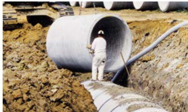
FIG. 9 Splay ended pipes being laid in a large radius curve. Jointed with E-Bands.
