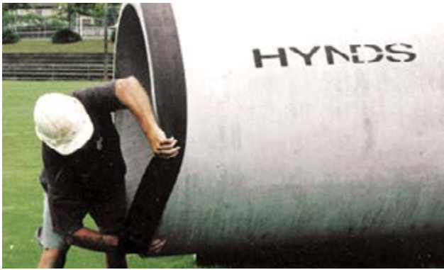
FIG. 5 E-Band is unfolded so that it is located midway between the adjacent pipes
