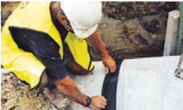
FIG. 7 E-Band is placed evenly around the pipe barrel in a fold
